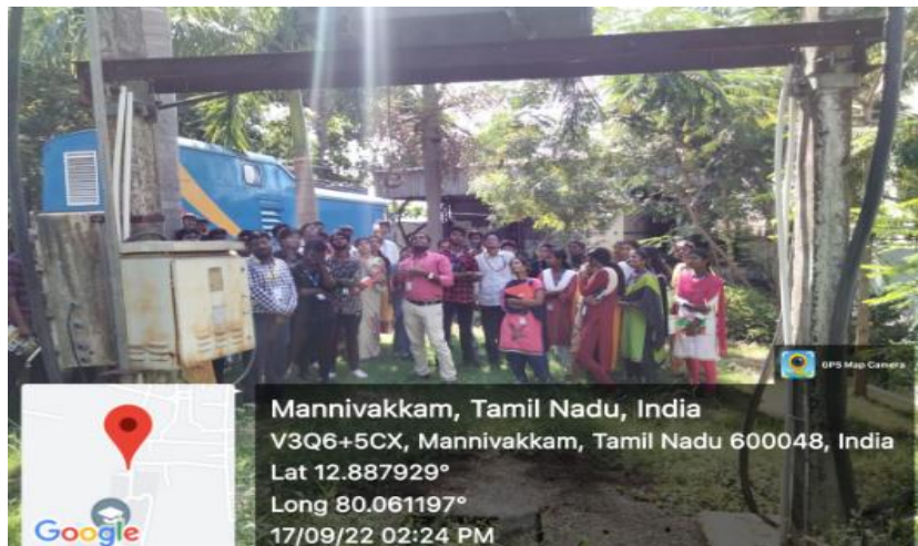
PERI Power transformers connections with HV/LT side
